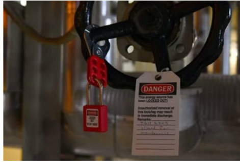
Figure 4.10 Lockout and tagging system
