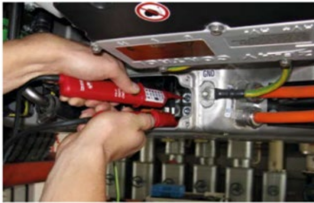
Figure 4.20 Checking residual electrical charges in the system
