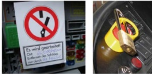
Figure 4.19 Measures to prevent reconnection
